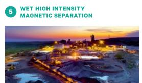
HMC is transferred from stockpiles by front-end loaders and fed to the Wet High Intensity Magnetic Separation (WHIMS) plant to separate magnetic from non-magnetic fractions.
